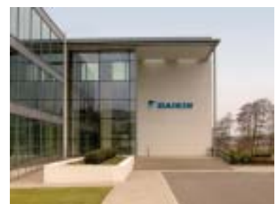
Daikin Airconditioning UK, Weybridge Head Office
